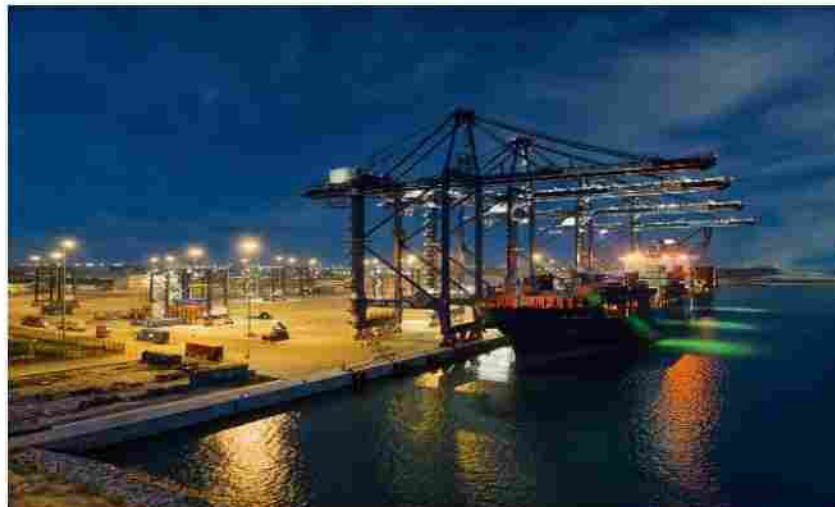
Lekki Deep Sea Port, integrated with the Lagos Free Zone
